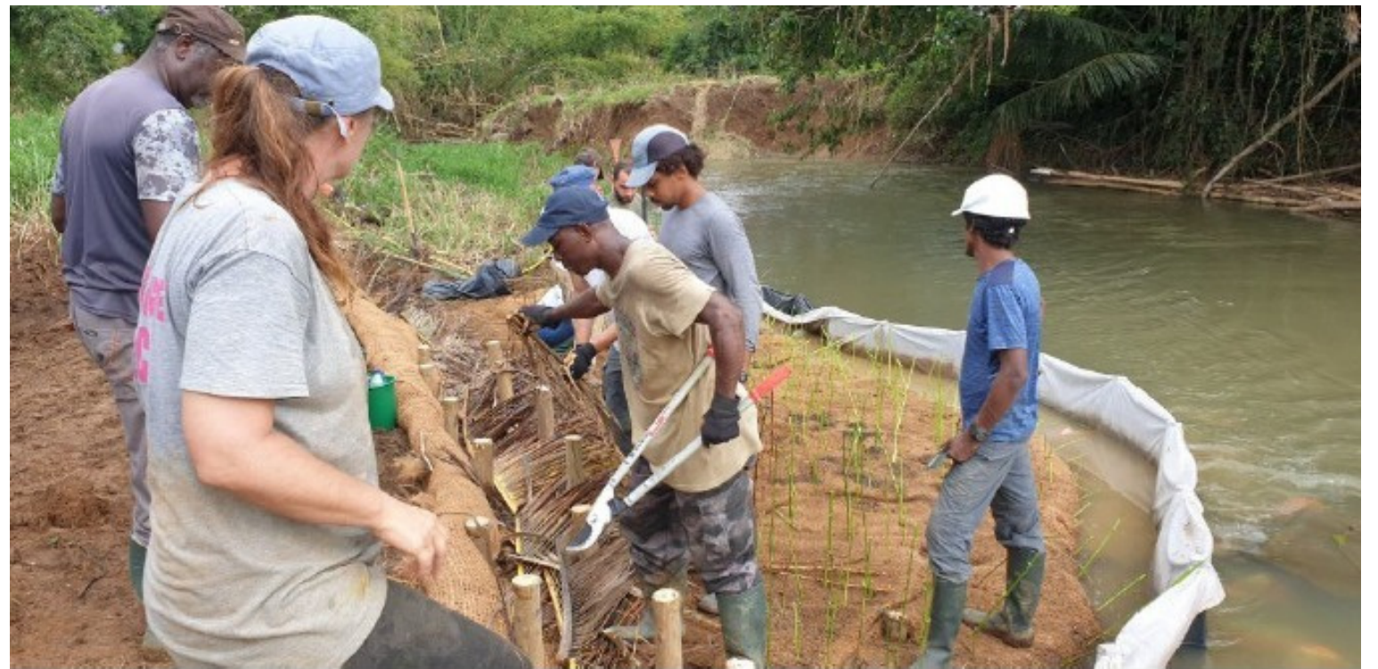
Illustration 9: Pose de la fascine
